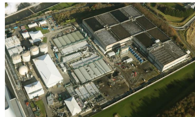
Ringsend Wastewater Treatment Plant
