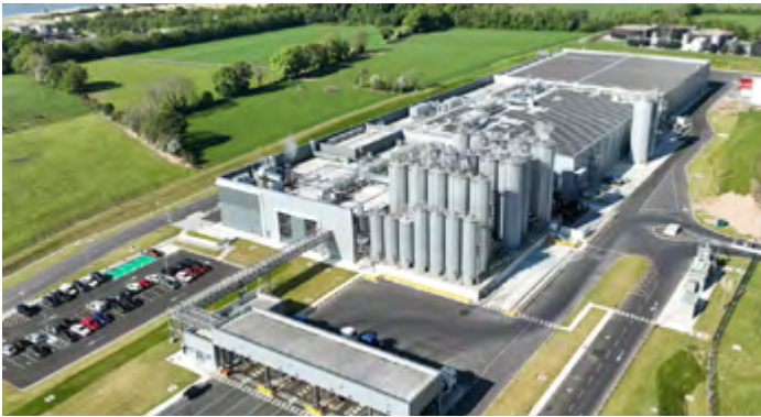
Overall view with wastewater treatment plant in the background
