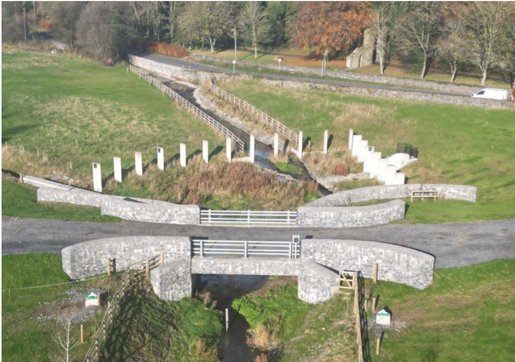
The vertical structures are precast columns which form part of the debris trap at the "defence line" of the scheme. The purpose of the columns is to trap any large floating debris / trees in a flood event and prevent them entering the flood relief channel.
